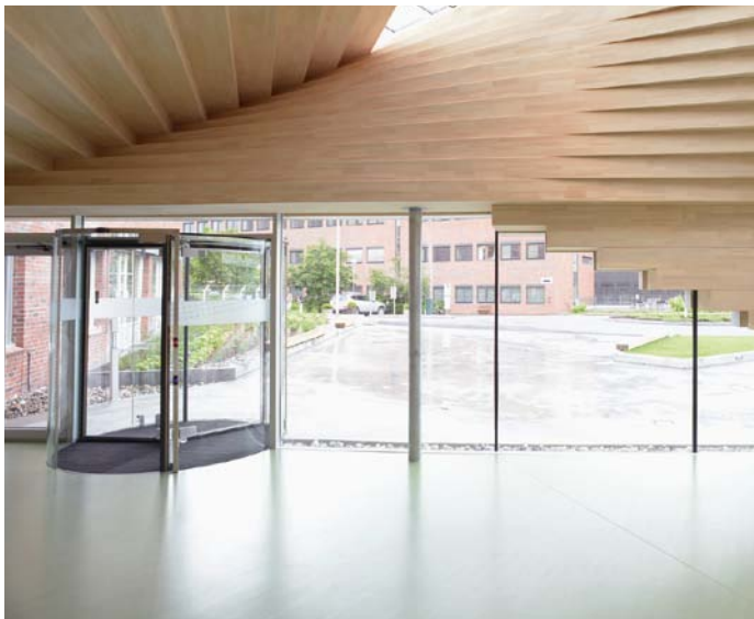
Drei Meter lange Grundelemente aus kreuzverleimtem Massivholz The basic elements are three metre-long, cross-laminated solid timber panels
