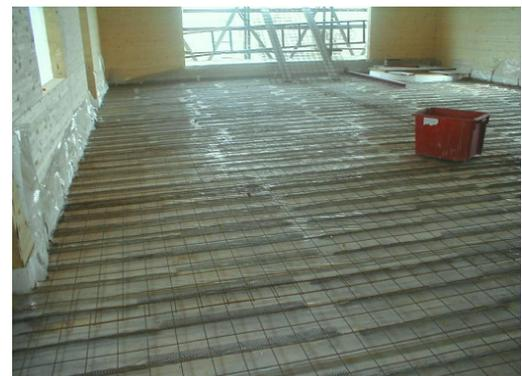
Glulam plate with HBV®-Shear Connector
